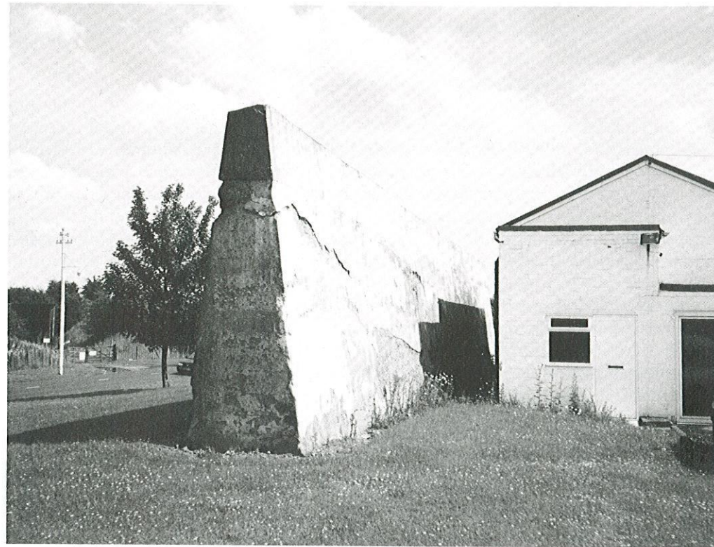
Thick concrete blast wall to protect surrounding buildings. 1999
